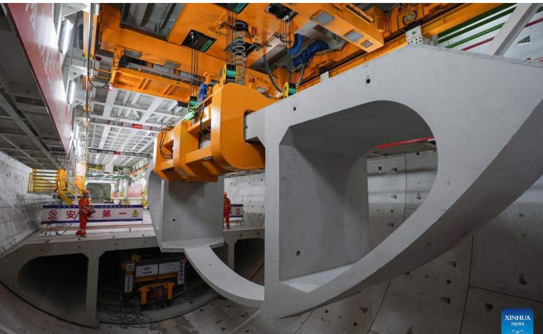
Technicians from China Railway 14th Bureau Group Co., Ltd. operate a crane inside the “Yongzhou” shield tunneling machine in the Jintang undersea tunnel of Ningbo-Zhoushan Railway in east China’s Zhejiang Province.
